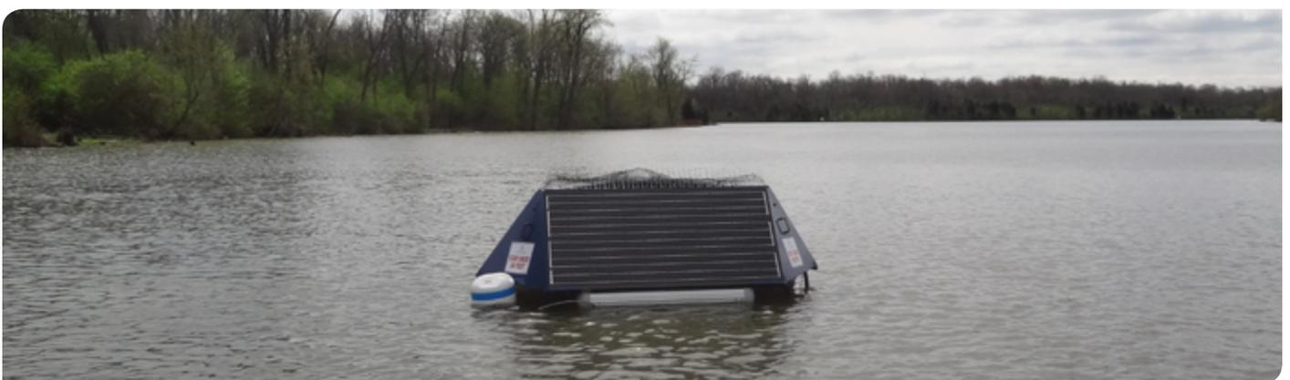
Figure 1: MPC-Buoy algae control system installed in Canoe Brook reservoir #1
