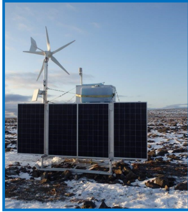
Permanent power source for a surveillance tower, North-West Territories, Canada Model: GC-Mobile
