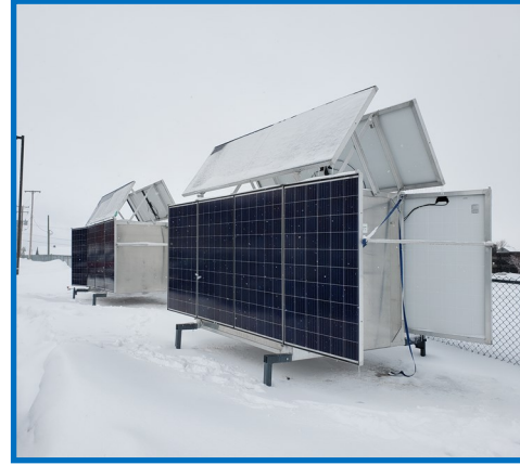
Solar energy system for a scientific research station in Quebec, Canada Two GC6— solar modules, with 3 kW solar power each
