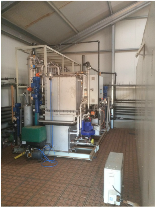
Biological Sewage Treatment
