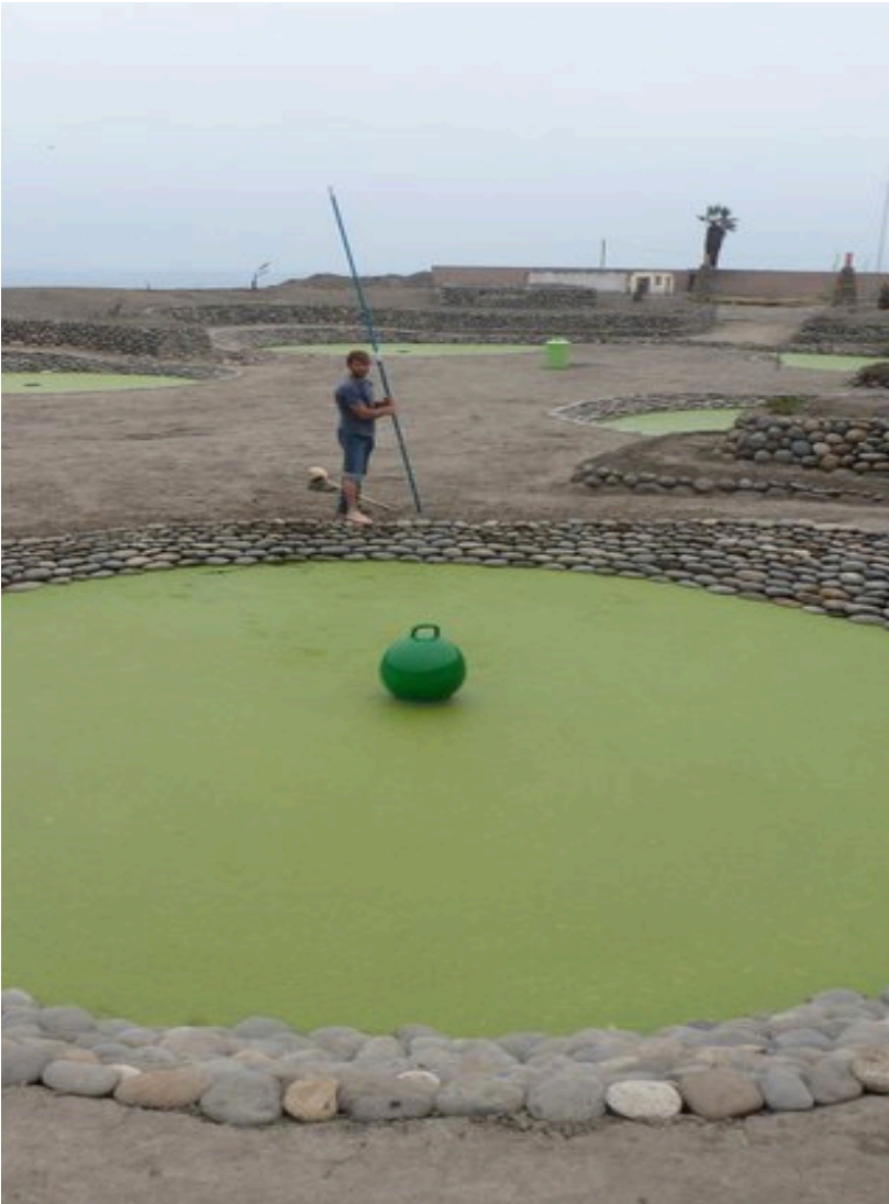
Barranca WWT Plant in Peru – Proven Technology
