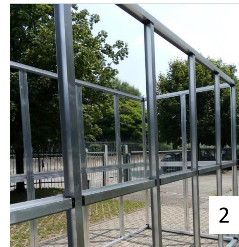
1 + 2) Basic frame details Omega profiles for height separation
