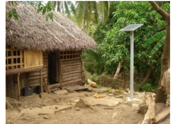
Solar Home System
