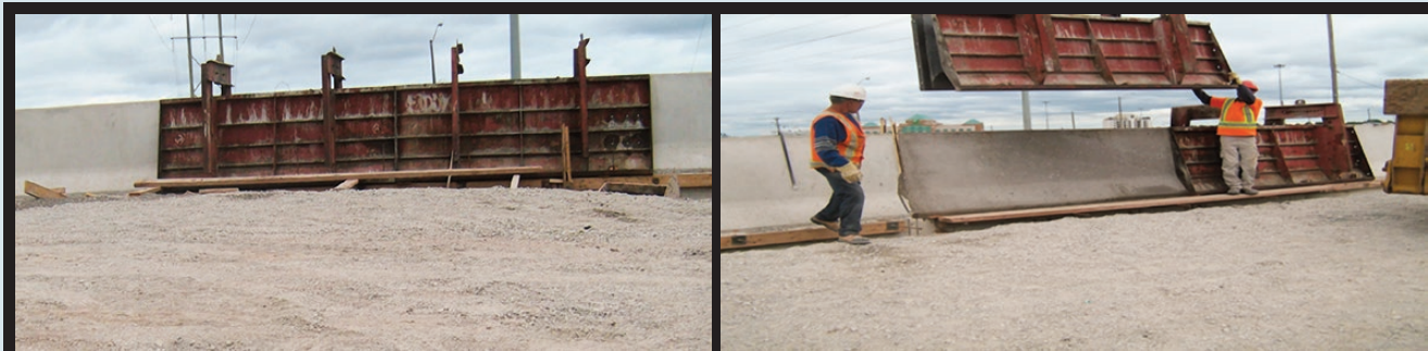
Figure 4. Bridge walls cured in less than two hours in subzero temperatures in Ontario, Canada. Credit: NanoArchitech.
