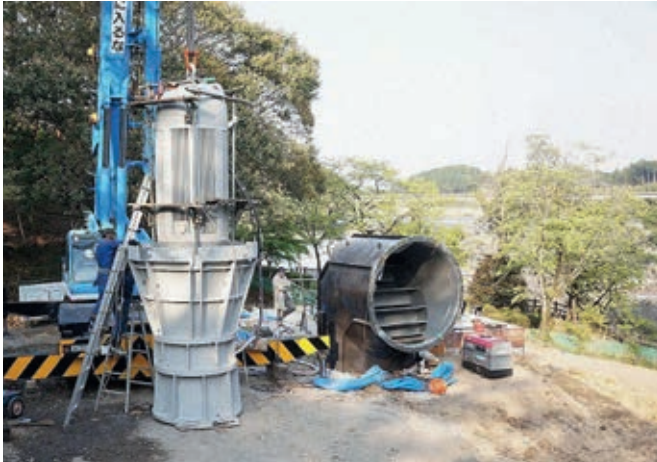
Bulb turbine ( Q = 5.5 \text{ m}^3/\text{s} , H_n = 11.5 \text{ m} , P_m = 495 \text{ kW} )
