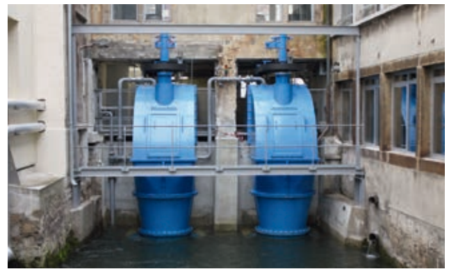
UMV plant in Vallorbe (CH), siphon-type turbines (Q = 5.0 m 3 /s, H n = 2 m, P m = 85 kW)
