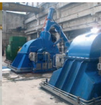
La Gorge turbines (F), horizontal axis, 2 nozzles (Q = 0.900 m 3 /s, Hn = 440 m, Pm = 3490 kW)
