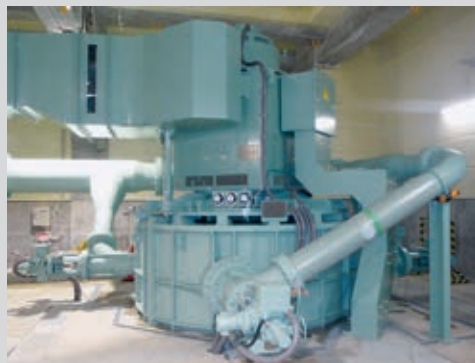
Makayabaru turbine (Japan), 3 nozzles (Q = 0.730 m 3 /s, Hn = 176 m, Pm = 1132 kW)
