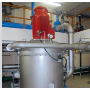
Haute-Pierre turbine (CH), 2 nozzles, back-pressure, integrated within a drinking water network (Q = 0.083 m 3 /s, Hn = 104 m, Pm = 76 kW)
