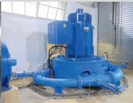
Lafarge turbine (F), 4 nozzles (Q = 0.590 m 3 /s, Hn = 85 m, Pm = 435 kW)
