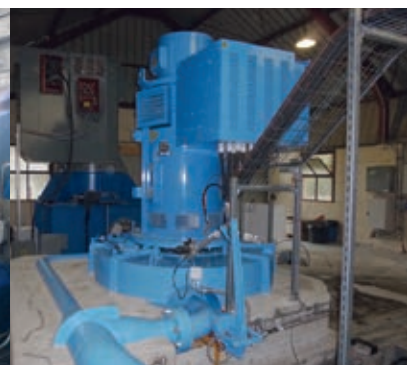
Lauzet turbine (F), 2 nozzles (Q = 0.186 m 3 /s, Hn = 271 m, Pm = 431 kW)
