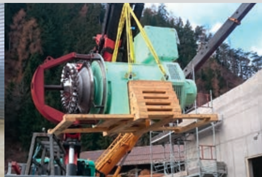
Torrents de Verbier turbine (CH), 4 nozzles (Q = 0.500 m 3 /s, Hn = 475 m, Pm = 2077 kW)
