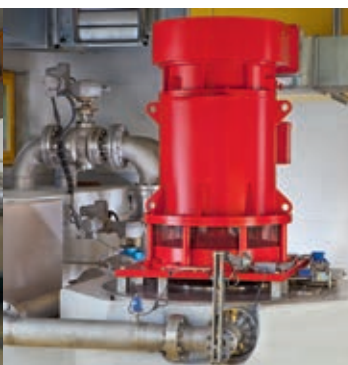
Profray turbine (CH), 2 nozzles, on raw waste water (Q = 0.100 m 3 /s, Hn = 430 m, Pm = 380 kW)
