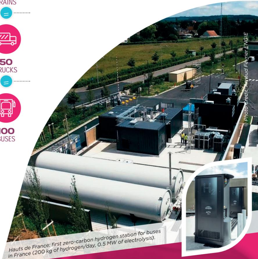
Hauts de France: first zero-carbon hydrogen station for buses in France (200 kg of hydrogen/day, 0,5 MW of electrolysis).
