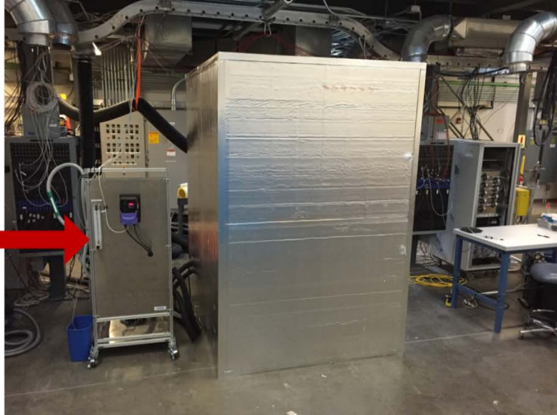
Figure 9. Calorimeter and pump station under test Photo by Eric Kozubal, NREL
