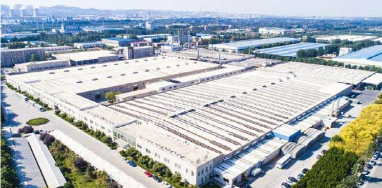
Shandong Factory I
