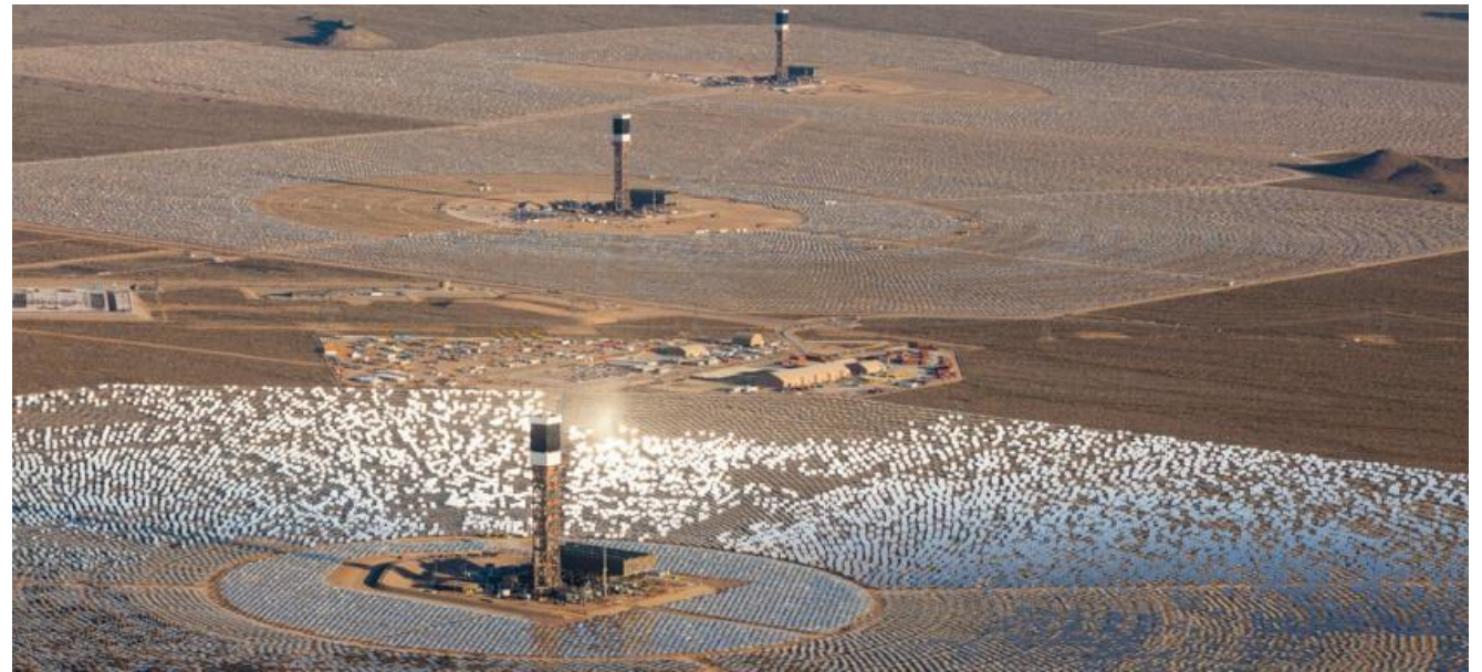
Ivanpah Solar Thermal Electric Generating Station, California, 377MW, $2.18 billion
