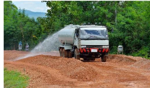
**2.** Add ECORoads to the water truck and spray ECORoads water solution onto the road base and windrow, as you would to bring soil to optimum moisture for compaction.
