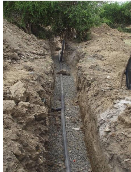
Clearford One™ ClearDigest™ Smart Digester™ (L) and Clearford One™ ClearConvey™ network of HDPE pipes (R) under construction
