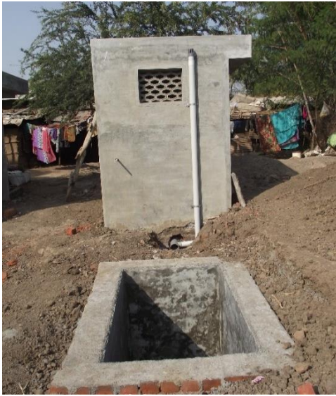
Clearford One™ ClearDigest™ Smart Digester™ (L) and Clearford One™ ClearConvey™ network of HDPE pipes (R) under construction
