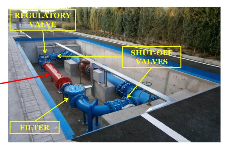
Parallel or bypass installation to the existing hydraulic facility, so in case of any contingency, water supply will be restored through the existing installation
