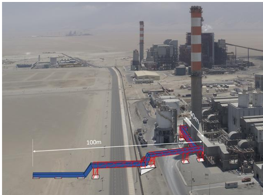
Flue Gas Pipeline Diverting Emissions from Stack to Carbon Farm Location
