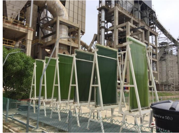
Argos: cement plant in Cartagena, Colombia
